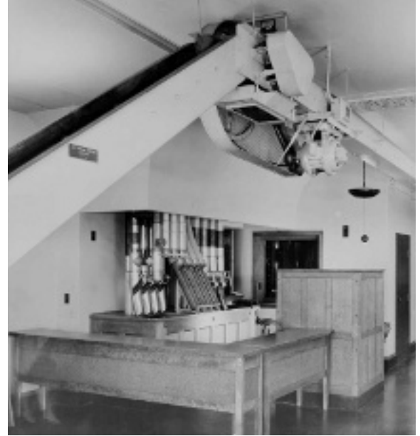
Mayo Clinic innovation in the Plummer Building, September 1930; Area in the "lower file" showing pneumatic tubes and vertical and horizontal conveyor systems used to move patient histories and other records throughout the buildings associated with medical practice.
